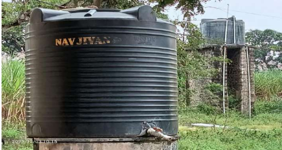
Water Tanks in College Campus
